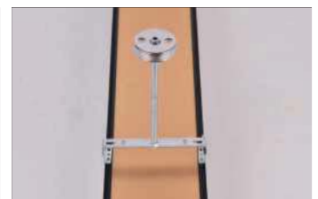
4. INSTALLATION CAN BE COMPLETED BY SCREWING THE SUSPENDER AND CONNECTOR. 4. 用螺絲將吊桿和連接器規定即可完成安裝
