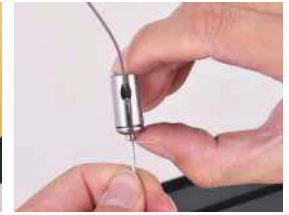
4.ADJUST THE LENGTH OF THE SUSPENSION LINES AS SHOWN. 4. 如圖調節吊線長度，完成安裝
