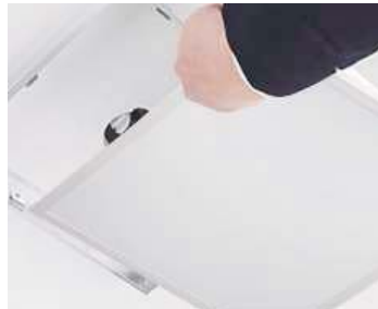
2. INTERNAL CONNECTION, CONFIRM THAT THE LAMP BODY IS BUCKLED INTO THE TRANSFER FRAME
