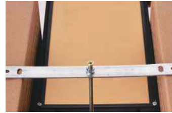
3.FANGTONG INSTALLATION COMPLETES BACK DISPLAY 3. 方通安裝完成背部展示
